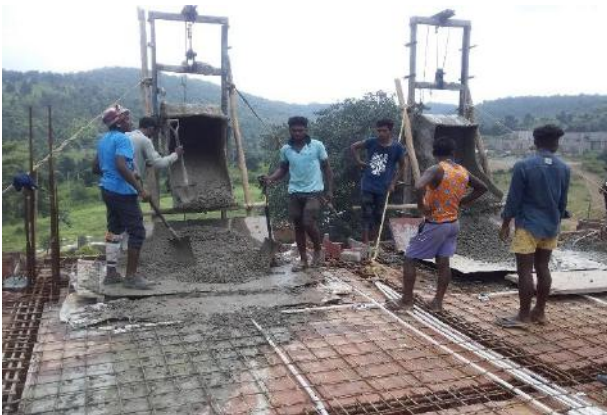
Fig.13(a) – Concrete placing by lift machine
