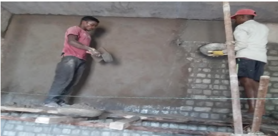
Fig14(a) – Plastering work
