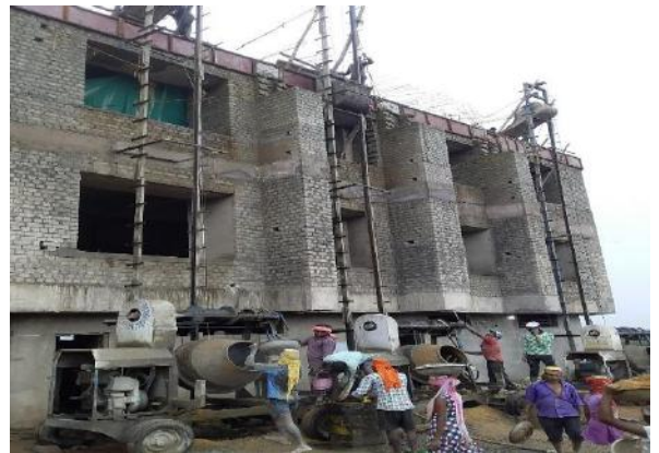
Fig.13(b) – Mixture machine & Lift machine set-up
