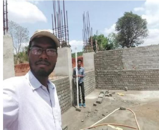
Fig.15(b) – Levelling staff on site
