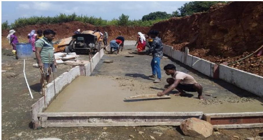
Fig.4(a) – PCC Work
