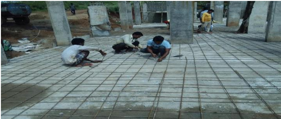
Fig.9 – RCC & PCC work
