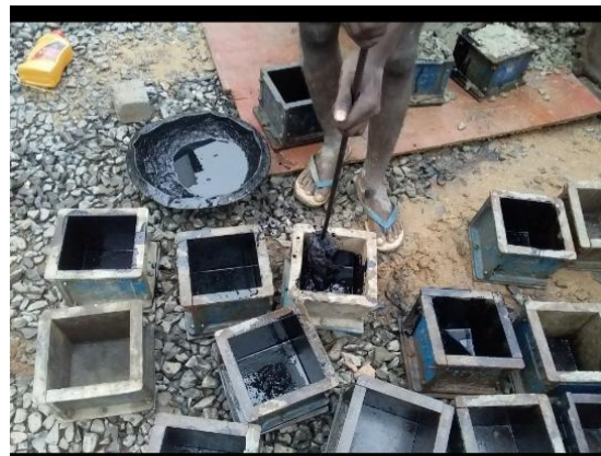
Fig.17(b) – Moulds after concrete is placed
