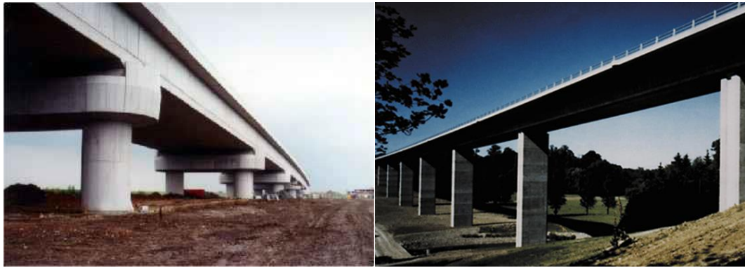
Figure 1. Concrete bridge structure
