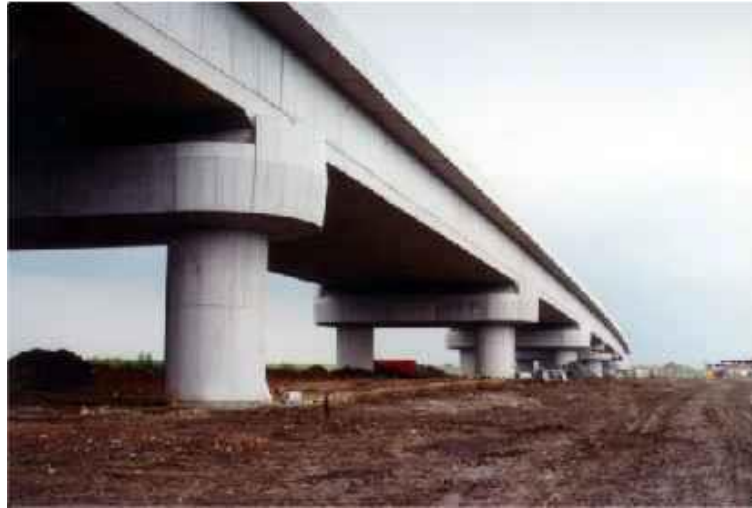
Figure 1. Concrete bridge structure
